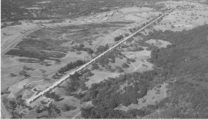
14. The 3-km- (2-mile-) long linear accelerator at the Stanford Linear Accelerator Center (SLAC). The electrons start off from an accelerator ‘gun’ where they are released from a heated filament, at the end of the machine at the bottom left of the picture. The electrons in effect surf along radio waves set up in a chain of 100,000 cylindrical copper ‘cavities’, about 12 cm in diameter. The machine is aligned to 0.5 mm along its complete length and situated in a tunnel 8 m below ground. The surface buildings that mark out the line of linac contain the klystrons which provide the radio waves.
